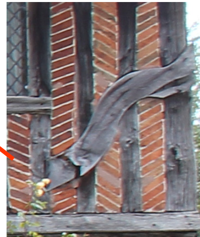
Fig 2: South east serpentine brace
