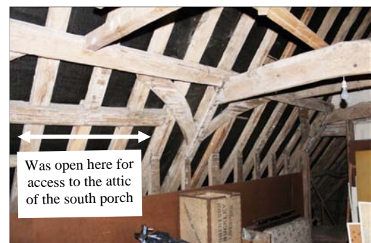
Fig 3: Roof over timber framed range
