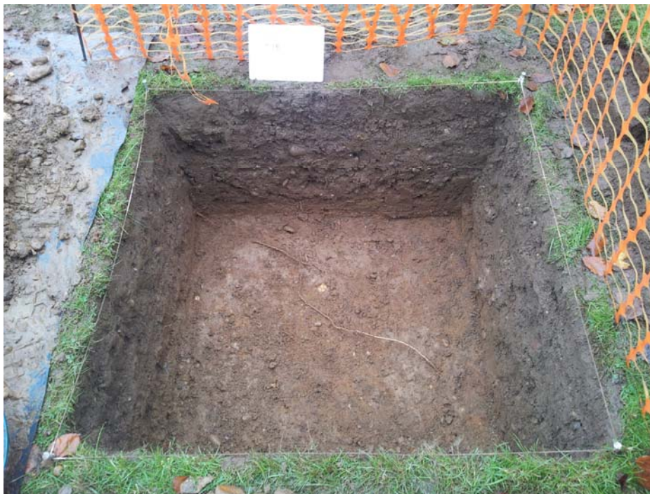
A completed pit
